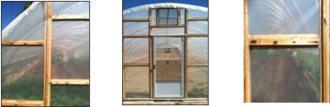
Figure 12 – Furring Strips on End Walls
