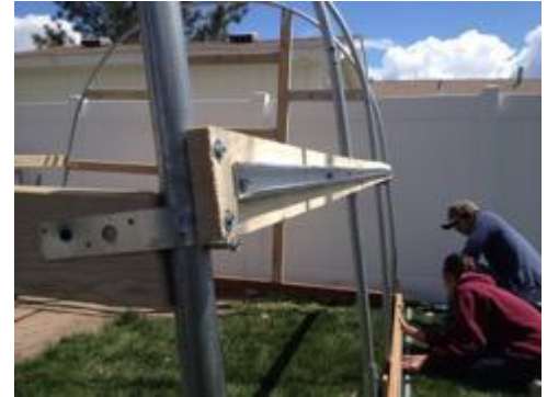
Figure 25 – Mounted Roll-Up Boards
