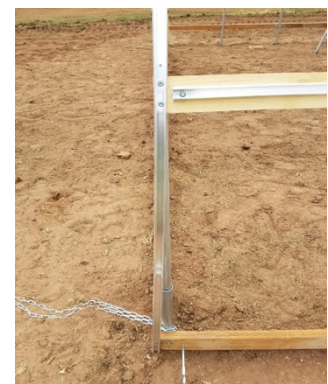
Figure 27 –U-Channel End Wall Attachment
