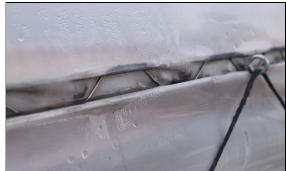
Figure 34 – Attaching the canopy.
