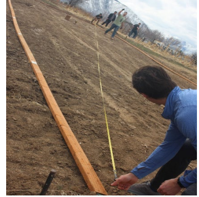
Figure 5 – Measuring diagonal corners
