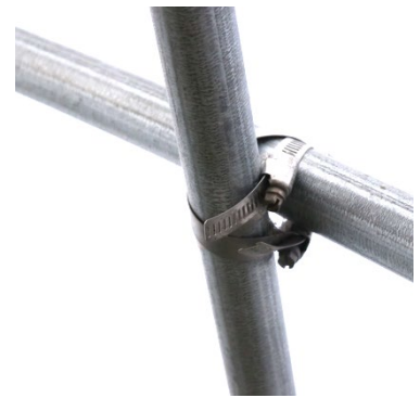
Figure 18 – Secure Purlin and Rib with Hose Clamps
