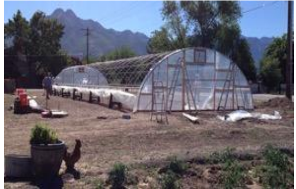
Figure 33 – Roll-Up Bars on the side of hightunnel
