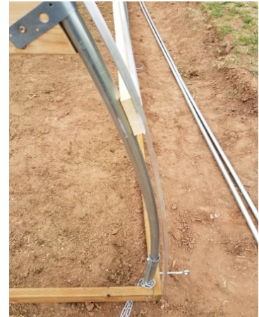
Figure 26 – Attaching U-Channel
