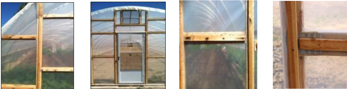
Figure 30 – Furring Strips on End Walls
