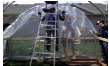
Figure 28 – Plastic on End-Wall
