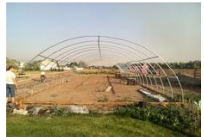
Figure 19 – Hightunnel with Purlins & Pipe finished
