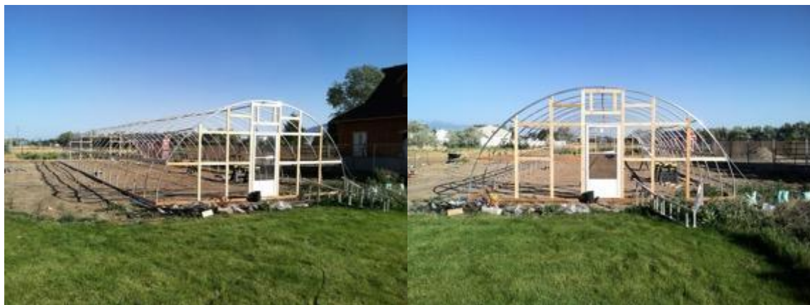
Figure 23 – Hightunnel with framing. Note opening for a bay door on back side (Right)
