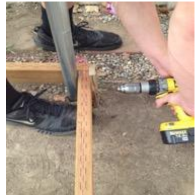
Figure 8 – Screwing stake to frame
