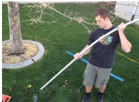
Figure 12 – Insert Ribs into frame Posts
