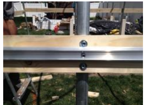
Figure 26 – Attaching Roll-Up-Board
