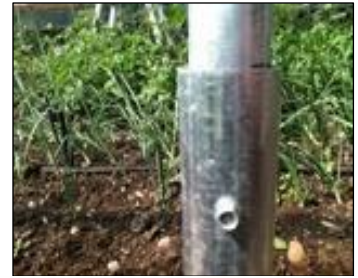
Figure 15 – Securing rib into post
