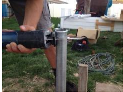
Figure 10 – Cutting off smashed post
