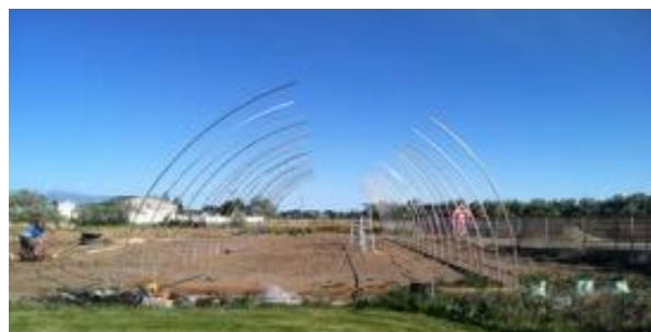
Figure 13 - Ribs hanging free waiting for joining
