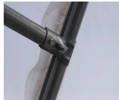
Figure 17 – Fasten End Ribs with T-end Clamp
